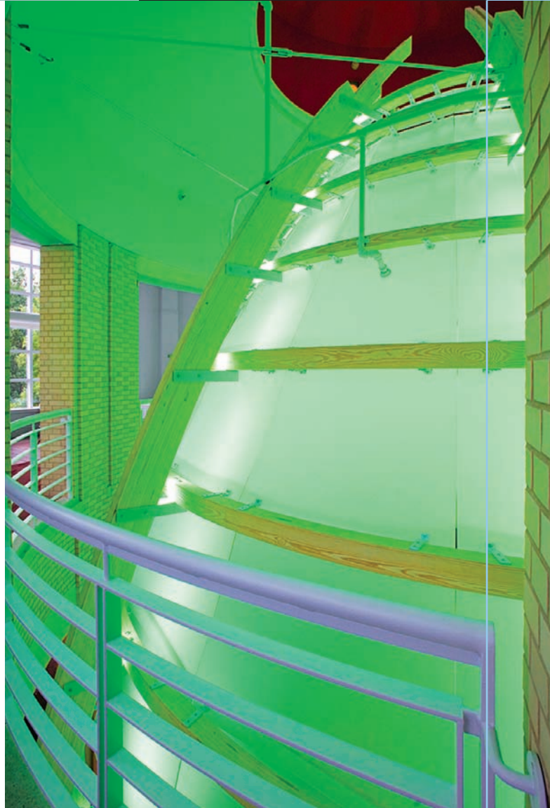
Laminate columns from Seech Industries are covered with translucent ‘eco-resin’ from 3form® (photo by Ed Massery).
